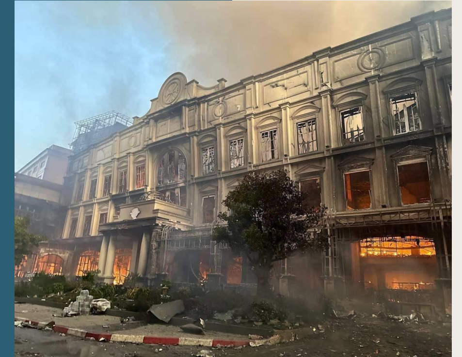
Severe Casino Fire in Poipet City, Banteay Meanchey Province, 28 December 2022
