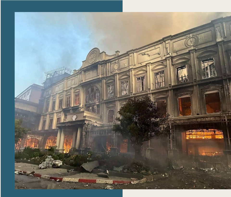
Severe Casino Fire in Poipet City, Banteay Meanchey Province, 28 December 2022
